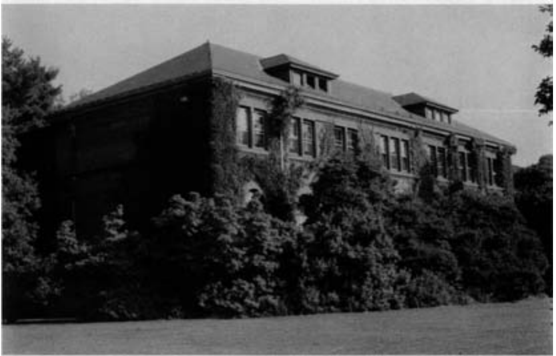
The Hunnewell Building in August 1992, a year before renovation. The several specimens of Magnolia stellata are over twenty feet tall and the Ilex pedunculosa over fifteen. The sheer mass of plants creates the impression of an overgrown foundation planting that completely masks the bottom two stories of the building.
